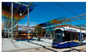
Tram stop in the center of the solarCity [Source: Mag. Stadt Linz, Archiv]
